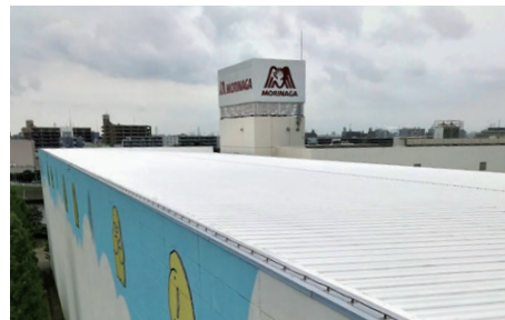
Tsurumi Factory: Thermal barrier-coated product warehouse roof
